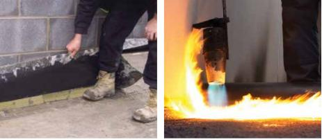
If applying a hot-melt bitumen membrane to a roof junction with a parapet wall using a flame torch, Marmox Thermoblock-PIR should be specified as this version is resistant to distortion which the standard block may experience if in contact with the flame gun. The PIR version has a slightly lower thermal conductivity (0.041W/ mK), is 53mm high and like the standard version a compressive strength of 9N/mm<sup>2</sup>.
